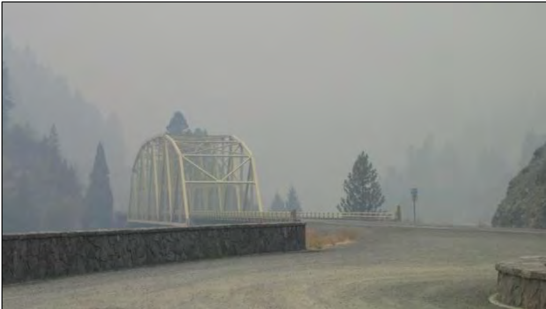
Figure 3.33. Smoke can obscure roads and bridges creating a public health and safety concern. Credit: ODF
