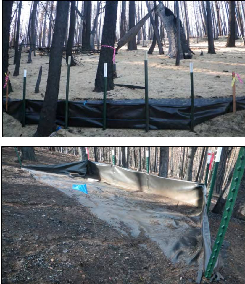
Figure 7.5. BAER installation of a sediment trap in a steep, high severity burn area. Credit: USFS.
